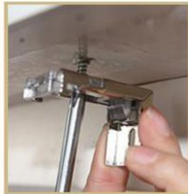
04. Fix the mounting hardware into the wall
